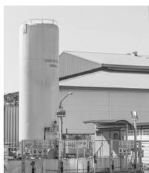
Bulk tanks are fixed tanks most commonly used to store large quantities of gas for transfilling into cylinders. They are generally found near the exterior of a building. Bulk tanks can also be placed on a distributor’s customer’s premises and leased to customers that utilize large quantities of gas in their operations. While bulk tanks can be moved, they are fixed when in use.
